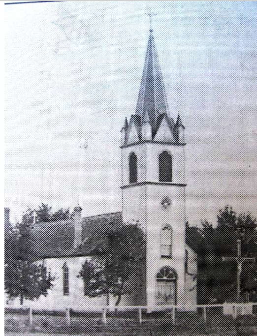
Sacred Heart Church, Flensburg, Original Structure
