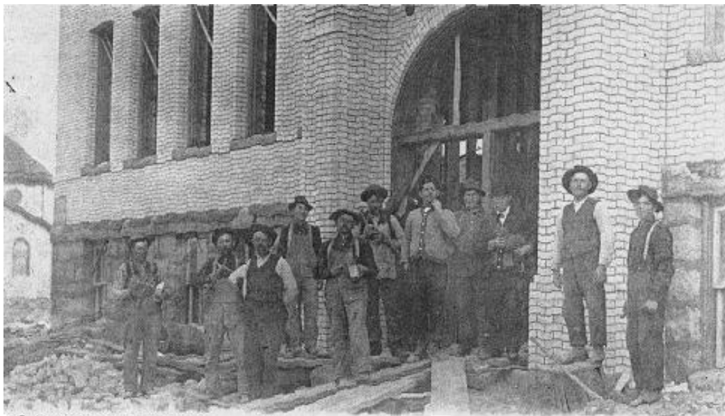
Photograph taken during the construction of the Gilman School (1909) From left: Bricklayer, George Kujawa, John Hep (the contractor), bricklayer, August Heir (?), bricklayer, Frank Kujawa, Walter Wojchiechowski (?), Paul Scyparski (church organist), John Zlock, Pete Kuzma Source: Benton County Historical Society
